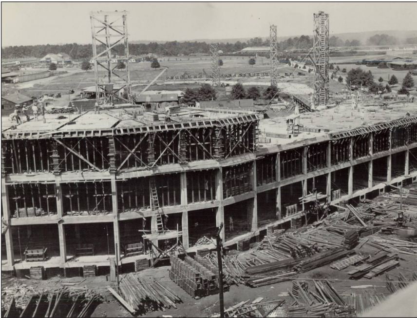
One of the three cuartels built between 1925-1935 is shown under construction.
