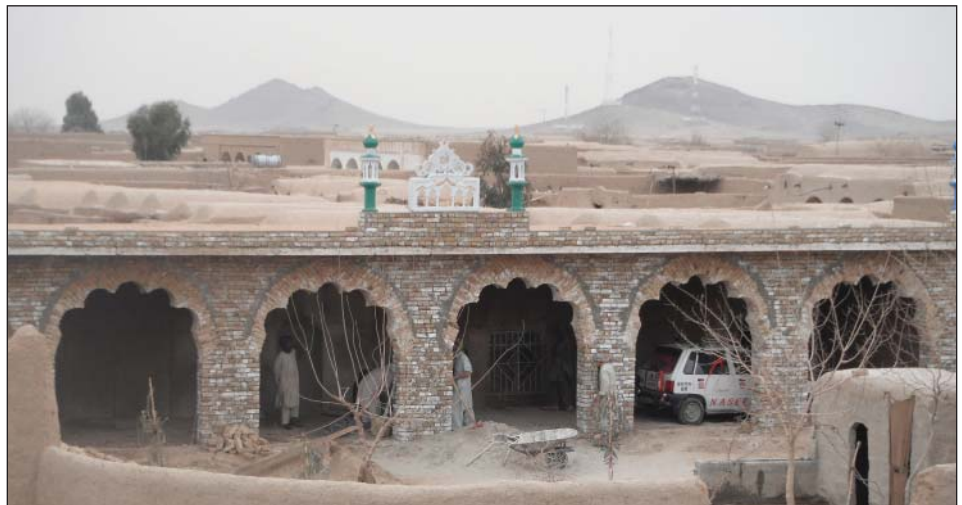
Local workers refurbish the mosque in Kandalay.
