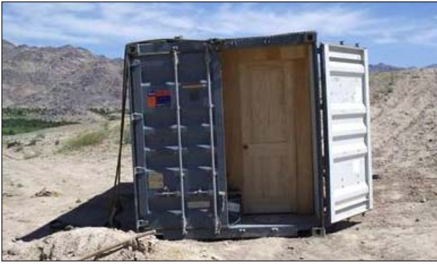
In terms of facilities, the author said the most valuable thing his unit did was to expand on the practice of turning connexes into small offices.
