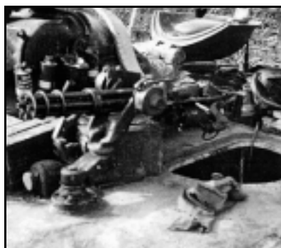
Above, at left, a 7.62mm Minigun salvaged from a helicopter was mounted in front of the loader's hatch... until the crew was ordered to remove it.
