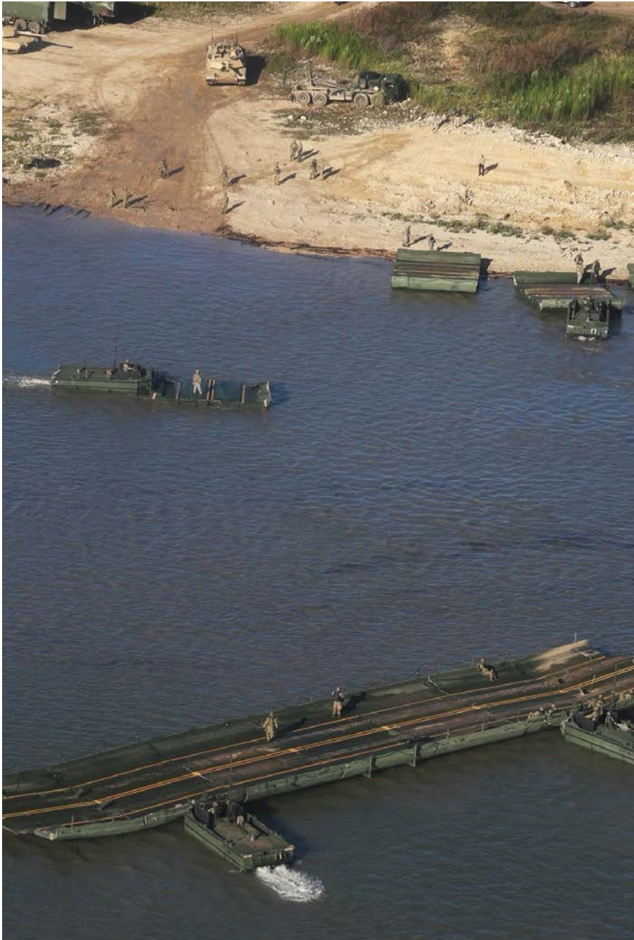
Figure 2. Multi-Role Bridge Company Raft Construction – The 43 rd and 74 th MRBCs assemble 7-Float rafts capable of ferrying multiple armored vehicles across Belton Lake. Early trips are conducted using a horizontal rafting style (pictured above), while subsequent iterations employ longitudinal rafting where the Bridge Erection Boats are positioned on both sides of the raft. (U.S. Army photo by MAJ Garrison Spencer, USACE Public Affairs Officer)
