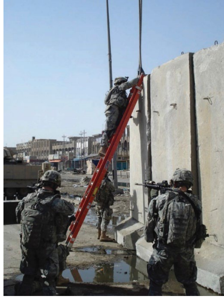
Figure 3. Infantry Soldiers emplace a section of T-wall.
