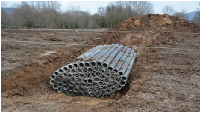
Figure 1. A Dutch pipe fascine emplaced in an anti-tank ditch.
