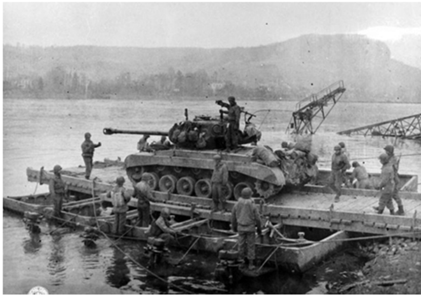
Figure 4. An M26 Pershing T26E3 from Company A, 14 th Tank Battalion, is transported aboard a pontoon ferry across the Rhine at Remagen March 12, 1945. The ferry was built by 1 st Engineer Heavy Pontoon Battalion. (U.S. Army Signal Corps photo)
