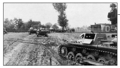
German armor employed in Norway was similar to these tanks photographed during the earlier invasion of Poland. Here, a Pzkpw I, foreground, acts as a command tank for the Pzkpw IIs in the background. Both light tanks, they were armed with machine guns and in the case of the Pzkpw II, a 20mm automatic cannon.
