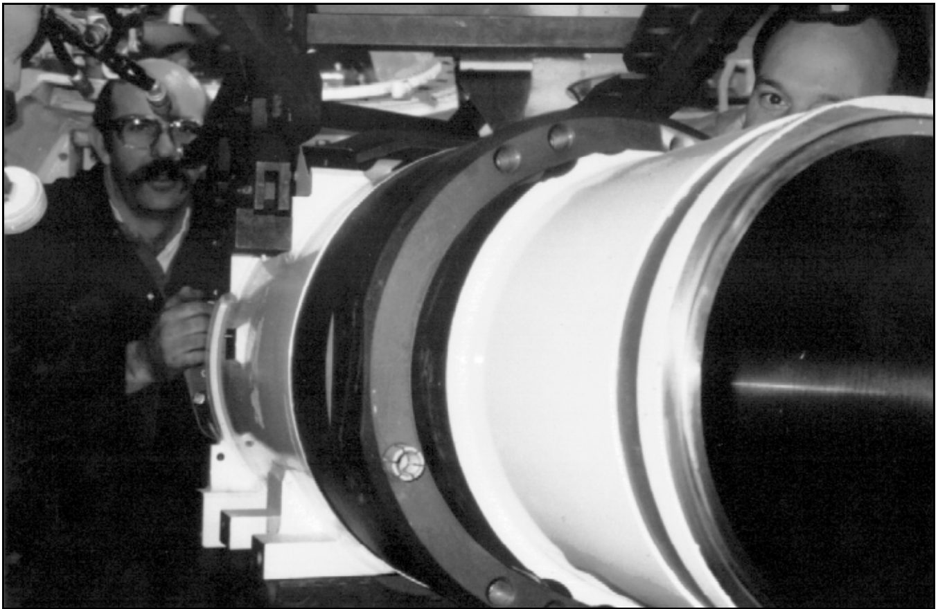
Technicians install a new gun mount within the tight confines of the Abrams turret. Below, crane lowers new mount into place.
