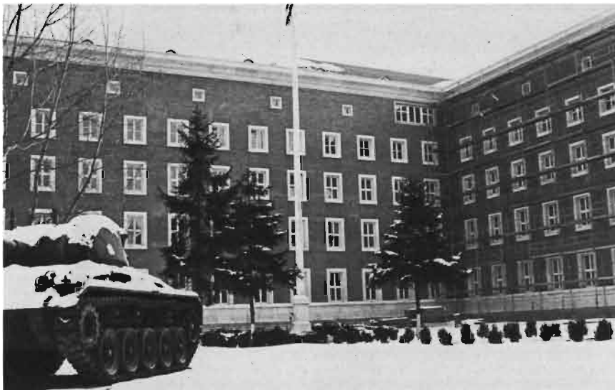
The shell-pocked exterior of the Merrell Barracks, damaged in WWII, is now being refurbished, one of the many improvements now being carried out by the Regiment.
