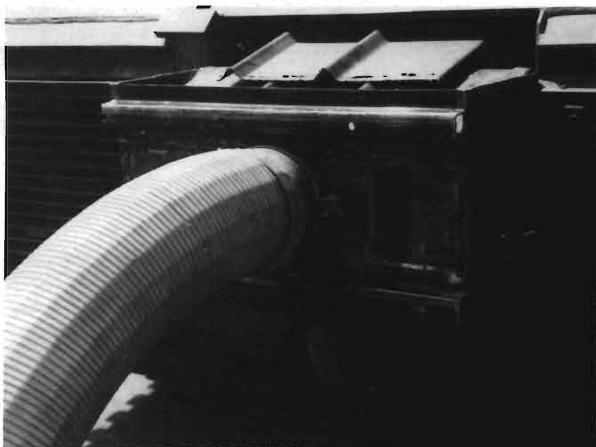
FIGURE 3. Closeup shows how Cannon Device is mounted on M1 grille.
